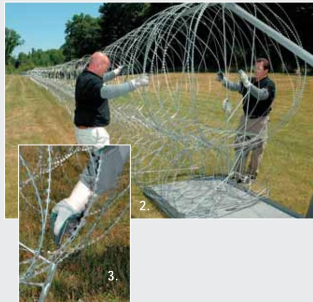
**2. STRETCH** Deploy the unit with a two man team. In just two minutes, a 480' triple strand barrier is in place.
